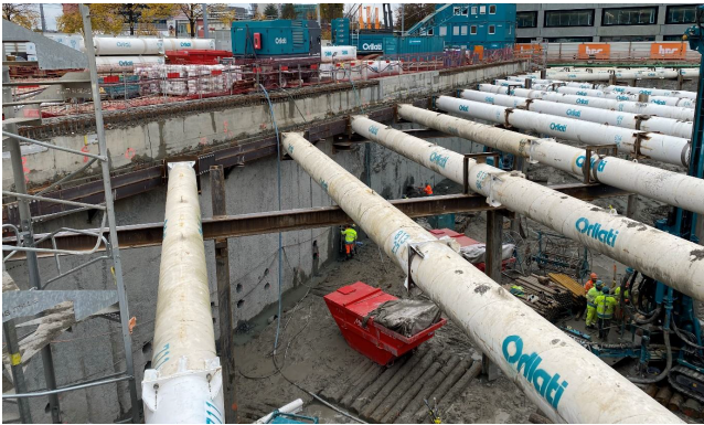
Figure 6: Picture showing stage 26 of the excavation.
